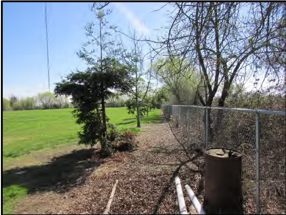
View of proposed easement to be acquired looking easterly from near existing pump station
