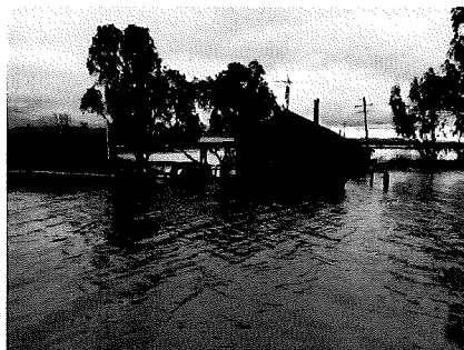
A building on Van Sickle Island in the Delta floods after a breached levee inundated the island with water. (Photo courtesy of John Sweeney)
